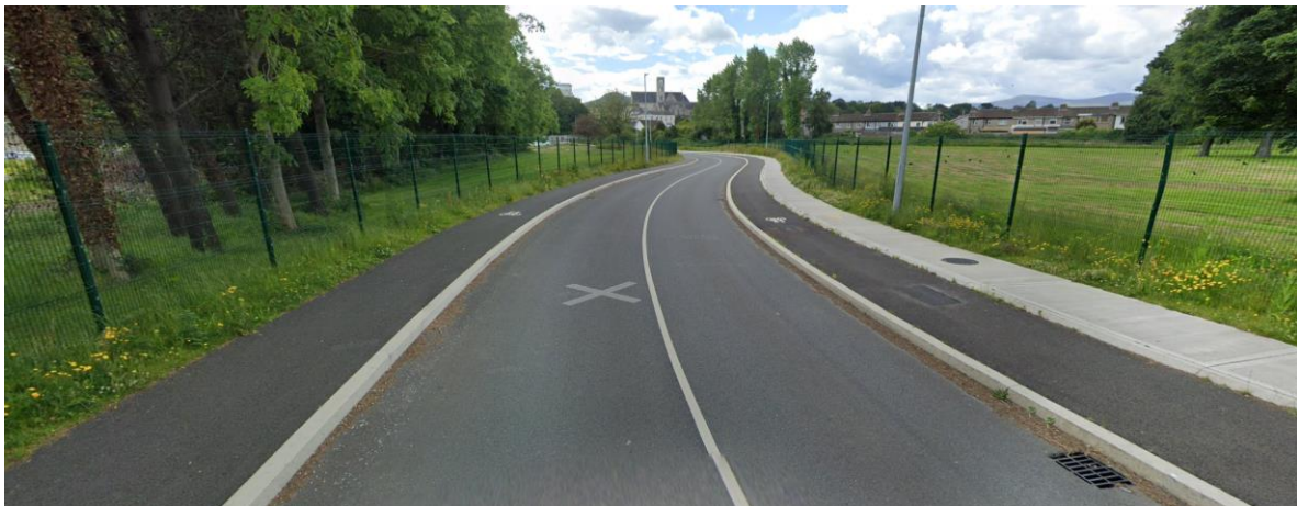
Figure 4-3 - Existing Southern Development Road
