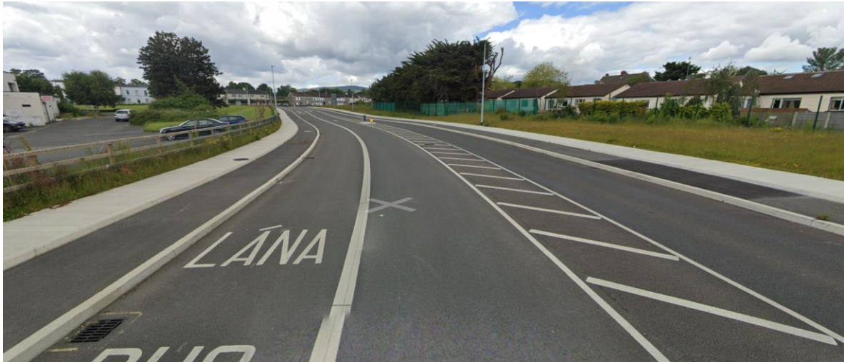
Figure 4-2 - Existing Northern Development Road
